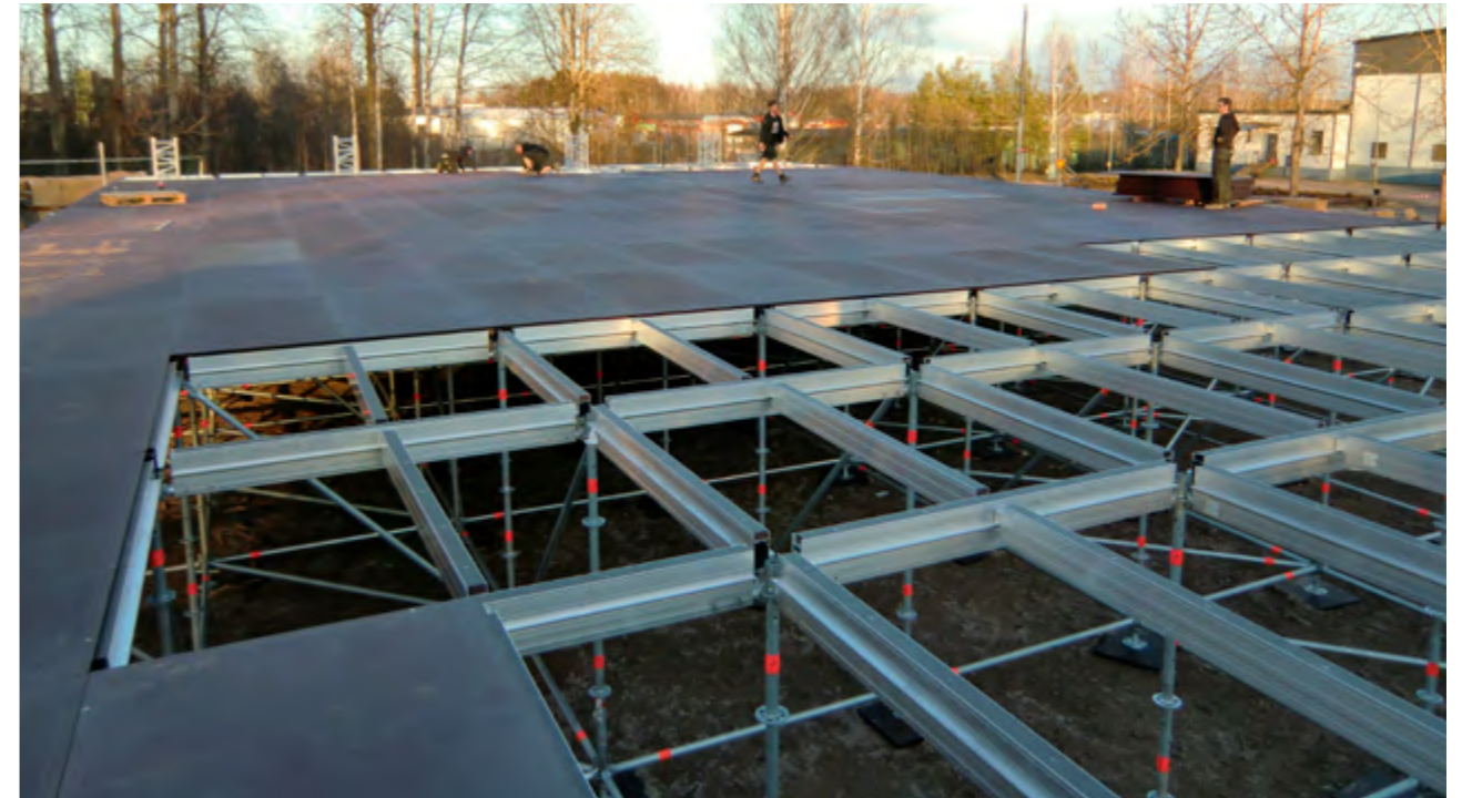
Photo: Prolyte Sales, Space Roof training Starlight
