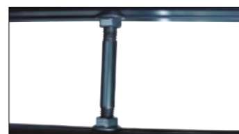
Fig 2. Connection of upper to lower profile by means of stud bolts which are fastened with a self locking nut.
